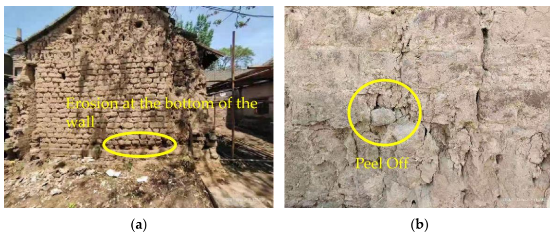
Figure 1. Disease map of cultural-relic buildings in western Henan: (a) erosion at the bottom of the wall; (b) peeling off the wall.
