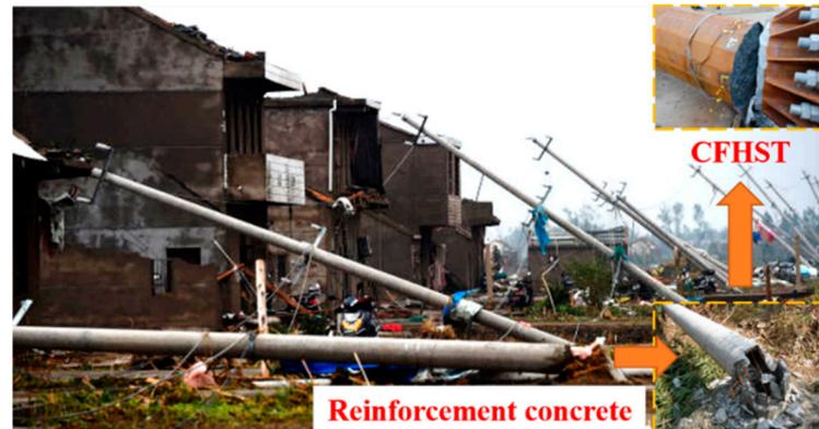
**Figure 1.** Transmission pole tower collapse.
