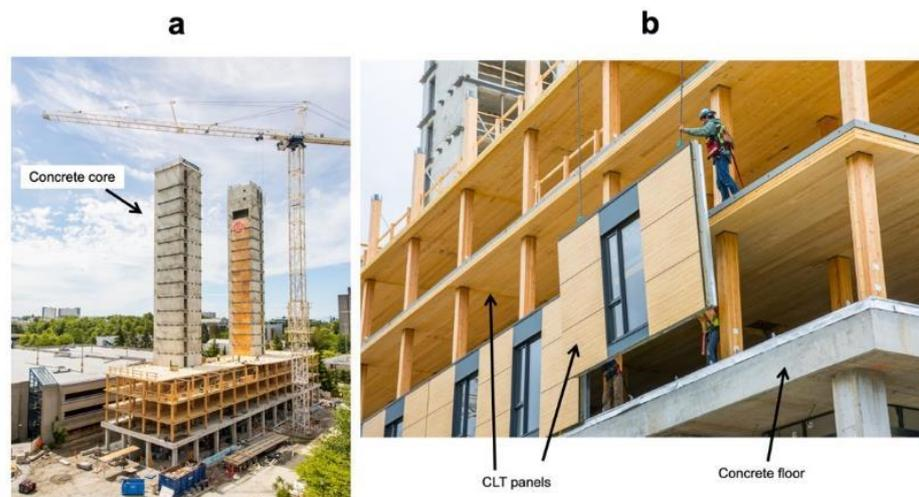
**Figure 6.** Brock Commons building progress: (a) concrete core and initial floor overview and (b) envelope cross laminated timber (CLT) panel installation. Modified from naturallywood.com; photographer: K.K. Law.
