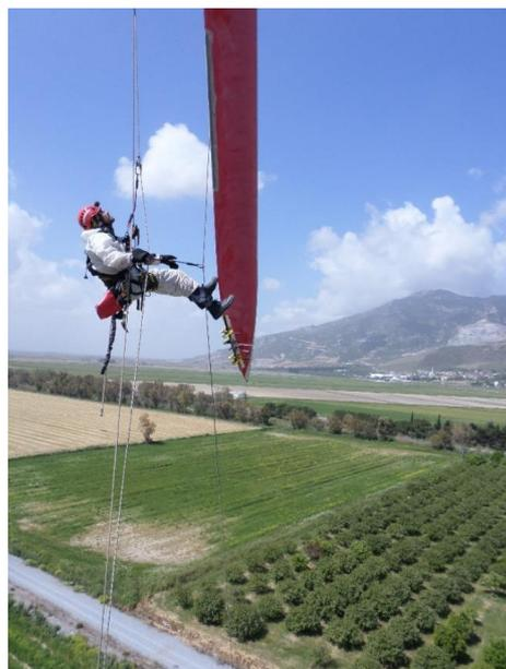
**Figure 3.** On-site repair of wind turbine blade. Reprinted with kind permission from Mira Rope Access, <http://www.mira-ra.com>, (accessed on 13 January 2021).
