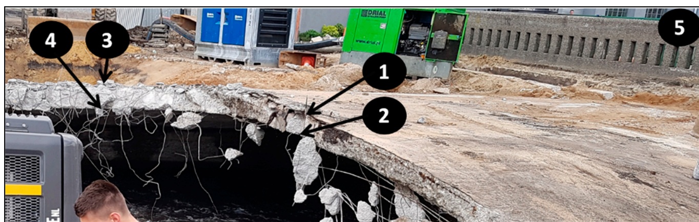
Figure 6. The RC (reinforced concrete) slab after removing the bituminous layer from the bridge.
