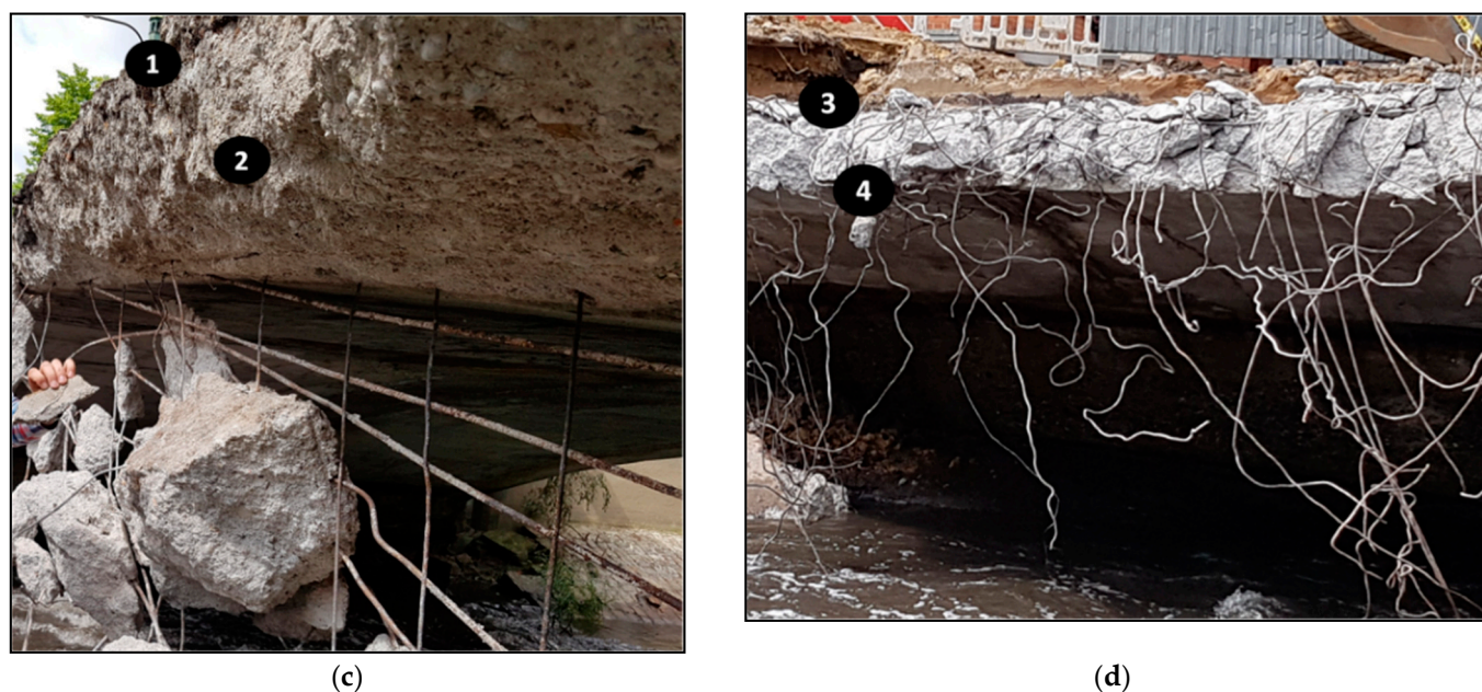
Figure 5. The sampling sites during demolition: Corroded steel mesh and carbonate icicles: (a) location of samples 2 and 4, (b) location of samples 2, (c) location of samples 1 and 2, (d) location of samples 3 and 4.
