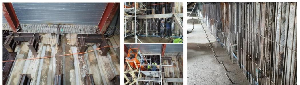
**Figure 2.** Examples of on-site waterproofing of pile walls (Dae-gu City, Korea).
