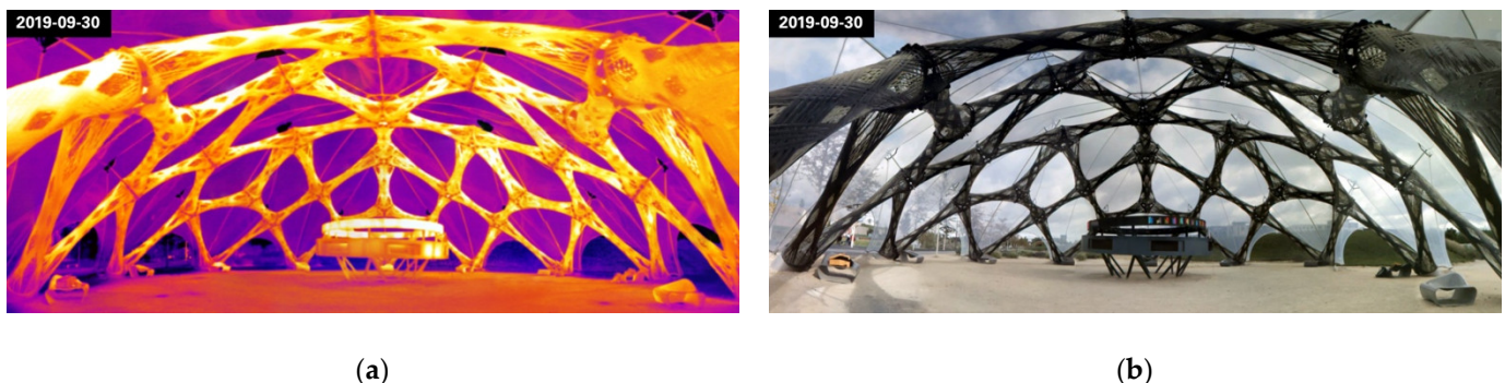
Figure 6. Stitched panoramic pictures of the BUGA Fiber Pavilion. Sun position towards the right side of the picture: (a) infrared spectrum (scale 10.0–23.0 °C); (b) visual spectrum.
