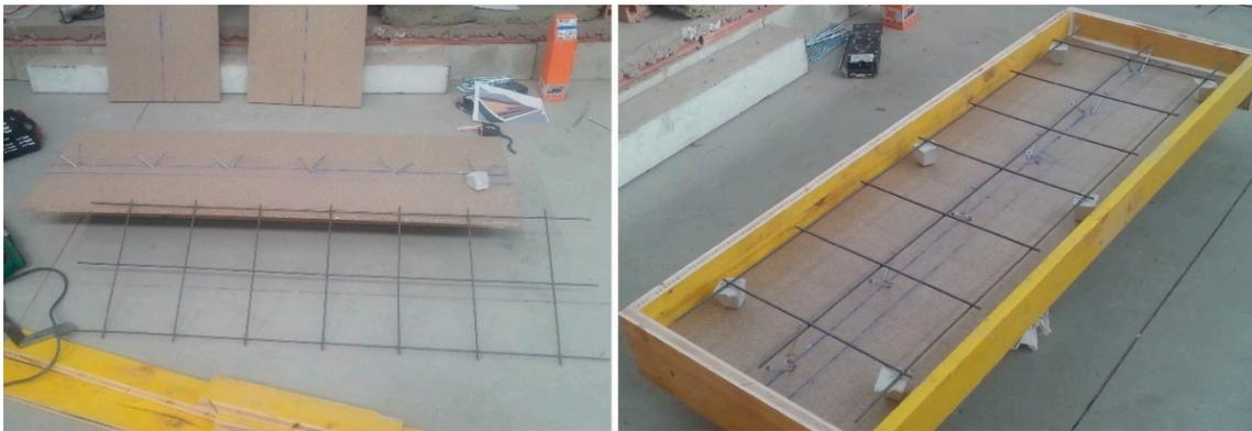
**Figure 5.** Final appearance of the mesh and formwork of the constructive unit.
