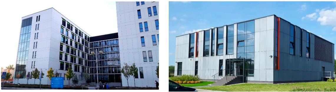
**Figure 1.** Exemplary uses of fibre-cement boards as ventilated façade cladding.
