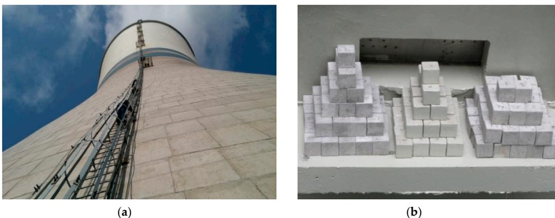
**Figure 2.** Auxiliary inspection facilities of the cooling tower. (a) Steel platform outside the tower; (b) concrete platform inside the tower.
