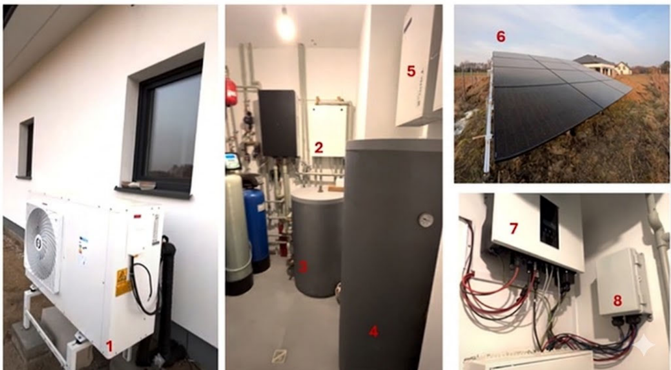
Figure 1. The main components of the installed hybrid energy system: (1) Monobloc HP outdoor unit; (2) HP indoor control unit; (3) DHW tank; (4) buffer tank; (5) BES; (6) PV installation; (7) inverter; (8) communication module.
