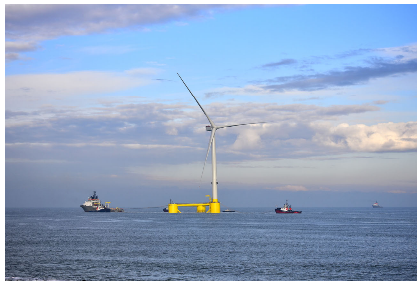
Figure 2. 9.5 MW turbine being towed to Scotland (photo courtesy of Principle Power) [12].
