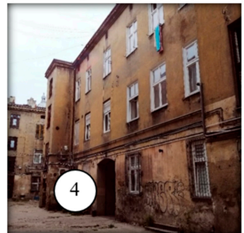
Measurement point no. 4 (view from the south).
