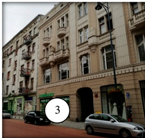
Measurement point no. 3 (view from the south).
