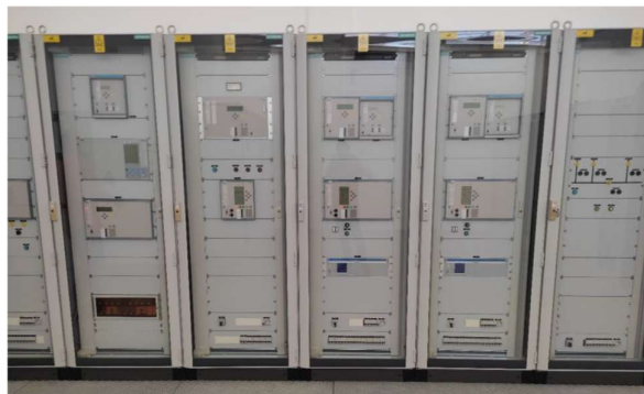
Figure 7. The São Martinho substation with starter batteries.
