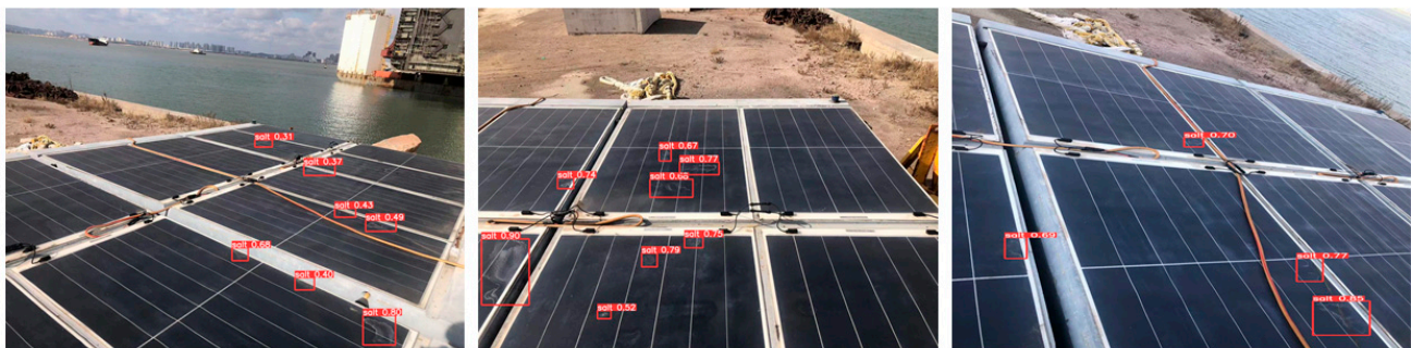
Figure 10. Detection results on actual offshore photovoltaic panels.
