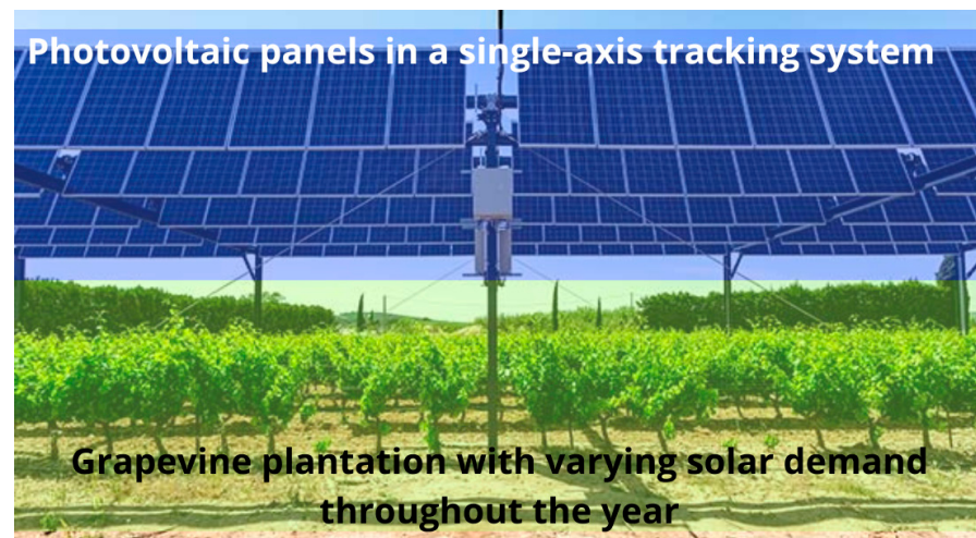
Figure 11. Sun' Anгри tracking agrophotovoltaic system in France. Source: own elaboration based on [93].
