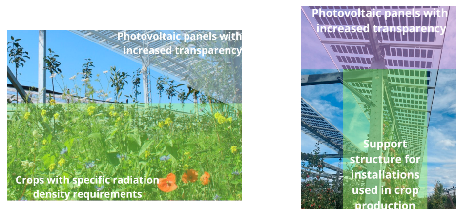
Figure 9. Use of double-sided photovoltaic modules. Source: own elaboration based on [81].
