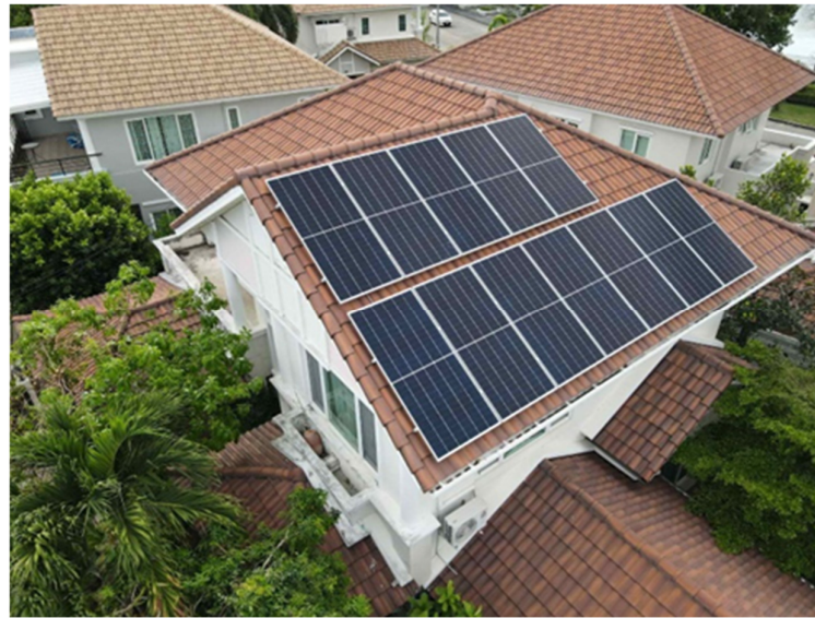
Figure 1. Solar rooftop installation of 5.5 kWp.
