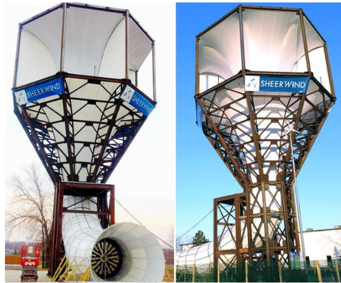
Figure 3. SheerWind's INVELOX tunnel-based wind turbine [4].
