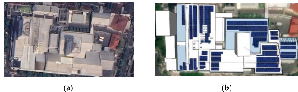
Figure 3. Depicts (a) the configuration of the FMCG facility in Indonesia and (b) the implementation of the rooftop solar power system.
