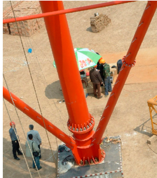
Figure 4. View of technical personnel undertaking field modal test.
