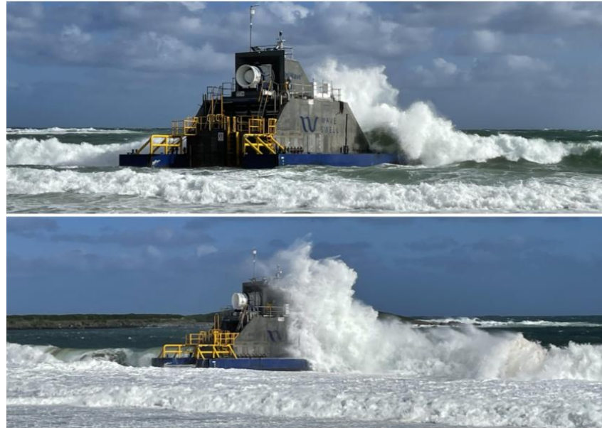
Figure 2. Large waves breaking and slamming into the Wave Swell Energy OWC WEC that was installed on King Island, Tasmania (photos courtesy of Assoc. Prof. Gregor MacFarlane).
