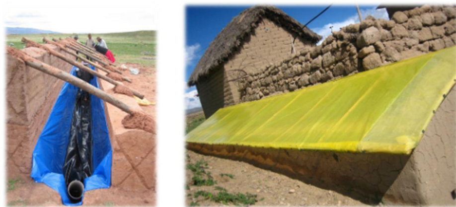
Figure 4. Open and closed trench for a tube digester in the Bolivian Altiplano [71].
