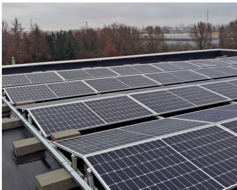
Figure 3. Appearance of a photovoltaic system with a peak power of 50 kWp placed on the roof of a university building.
