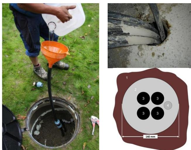
**Figure 7.** Left: procedure for injection of PCM into BHEs; top right: photo of a completed BHE; bottom right: section of a BHE. 1—ground, 2—borehole (space for grout), 3—BHE tubes, 4—injection tube [20].
