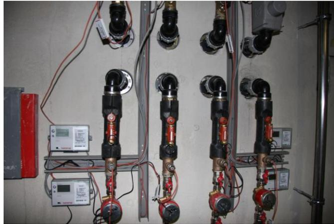
**Figure 8.** BHE inlets and outlets after the installation of the heat meters [20].
