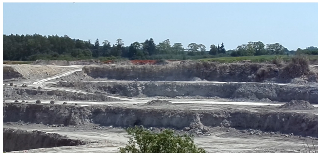
Figure 3. Blasting works at open-pit mine.
