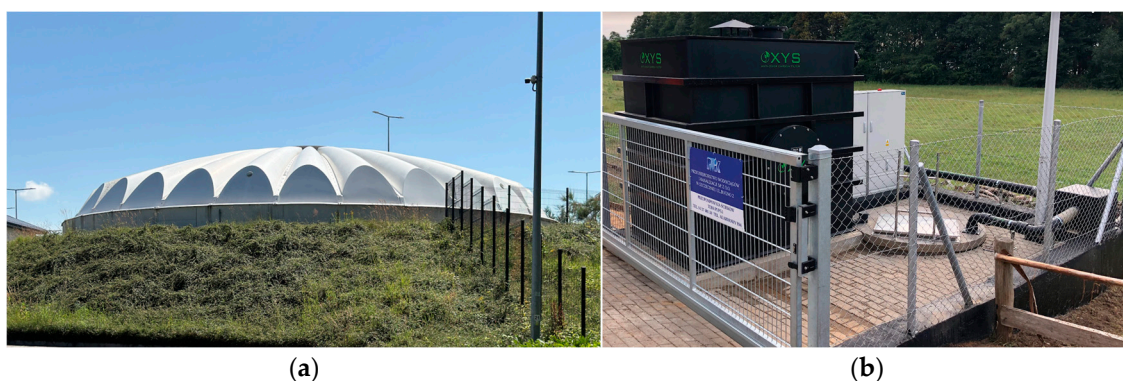
Figure 1. Example of encapsulation of a secondary settling tank in a municipal wastewater treatment plant (a) and elimination of odors from the expansion well of the wastewater system by adsorption on activated carbon (b) (own photo).
