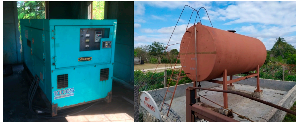
Figure 4. (left): The engine-drive AC generator operating in Guasasa; (right): diesel tank of the generator set in Guasasa (source: authors).
