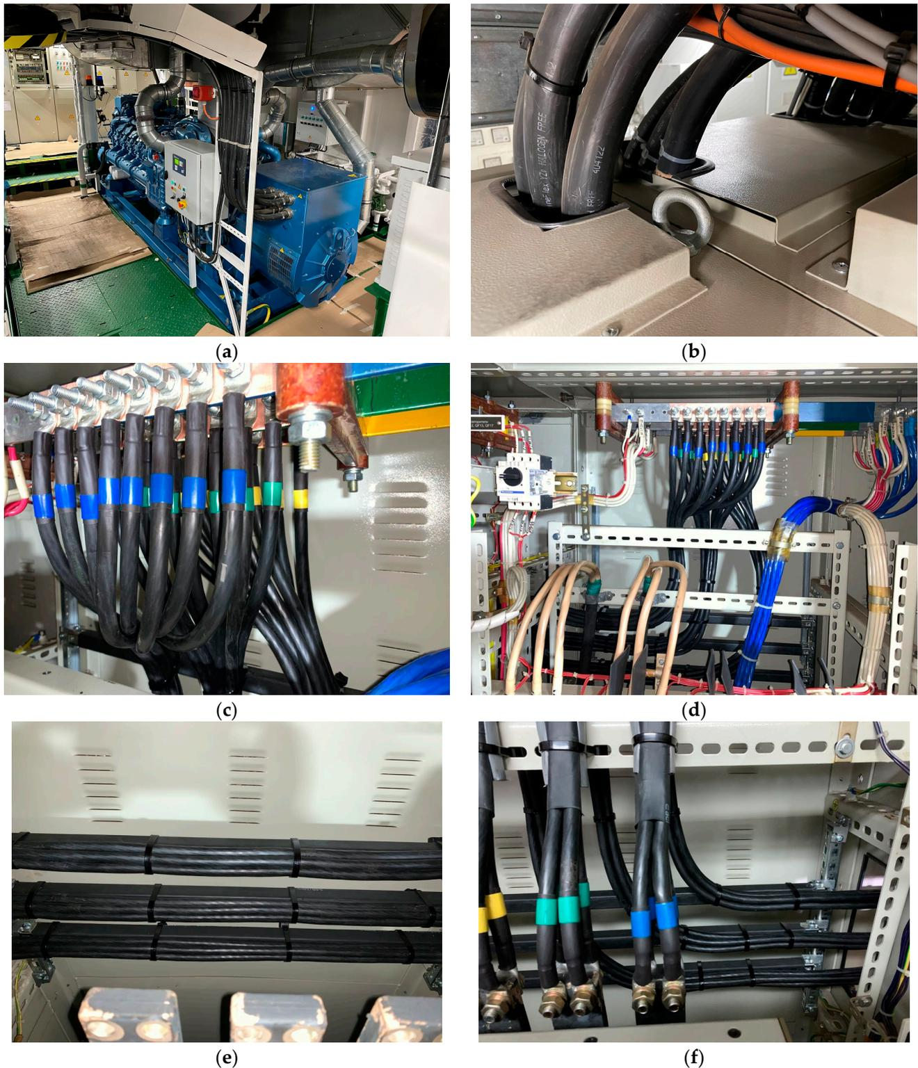
**Figure 4.** Installation methods and types of connection of cable lines: connection of cable line to SG (a) and UR (b), connection to MSWB (c,d), laying out the SCL at vessel (e,f).
