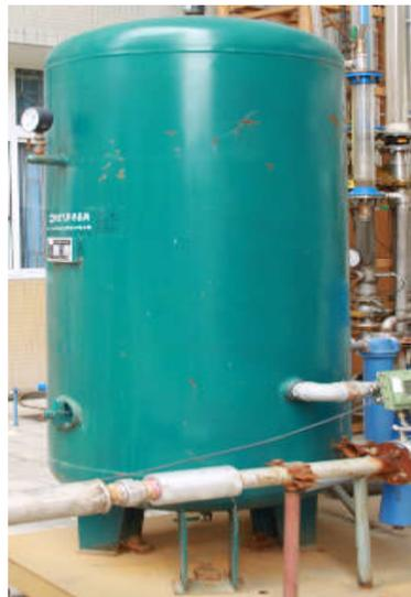
Figure 9. Gas storage tank.
