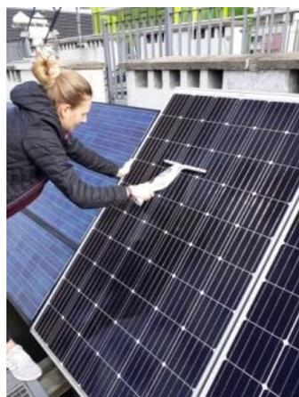
**Figure 2.** Collecting contaminants from the module with a vacuum cleaner (photo by J. Teneta).
