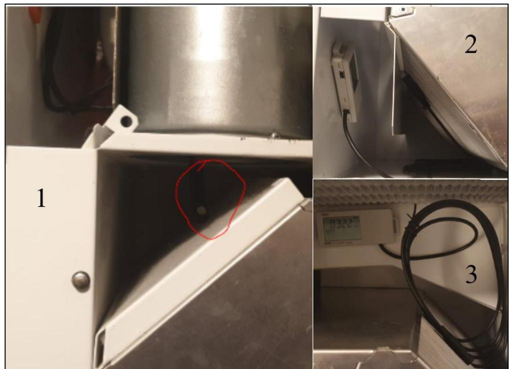
**Figure 2.** Placement of temperature—humidity sensors in the ventilation equipment. 1—exhaust air, 2—supply air, 3—outside air.
