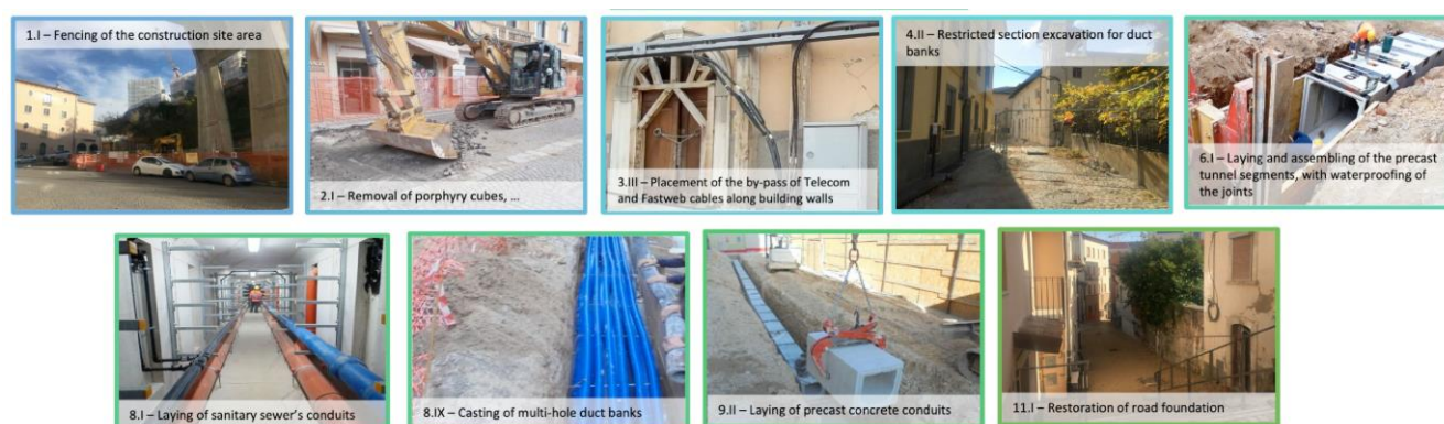
Figure 4. Detailed work phasing for the realization of the utility smart tunnel in L'Aquila. Thirteen working phases have been identified and each of them was subdivided in sub-phases (or activities). These phases stretch from the construction site set-up (phase n. 1) to its dismantling (phase n. 13). In the figure, photographic documentation of some of the sub-phases has been provided. The coordination between this construction plan and the site subdivision strategy allowed for parallel execution of the work (Figure 5) to reduce the project duration and reduce the laydown areas. At the same time, the adoption of the prefabricated elements further sped up the process, reducing the on-site energy demand with a lower impact on the urban environment.
