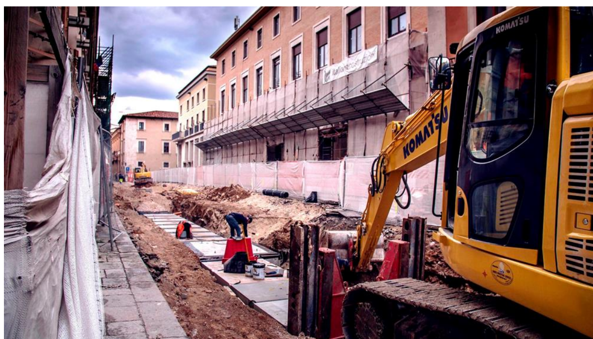
Figure 2. Positioning and assembly of the prefabricated elements to host the utility networks along Corso Vittorio Emanuele in L'Aquila.
