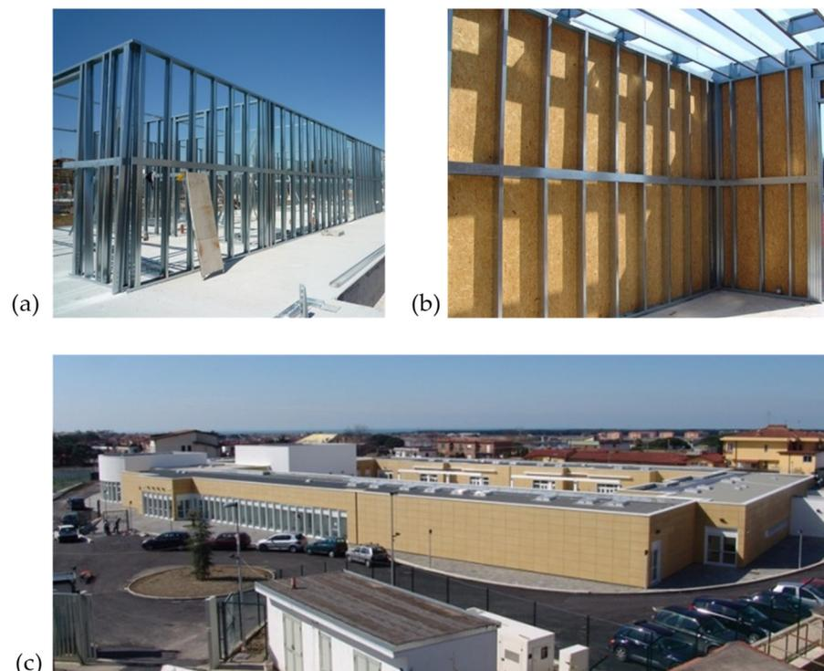
**Figure 1.** CFS school construction process: (a) CFS structural walls, (b) Sheathing of CFS walls, and construction of the roof, (c) Finishing and final result.
