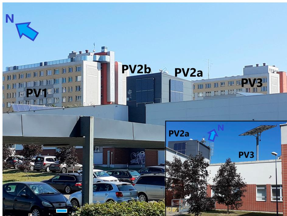
**Figure 2.** General view of the hybrid power plant, PV1—a fixed-tilt system with optimally directed panels, PV2a and PV2b—the panels on the facades, PV3—a solar tracking system.
