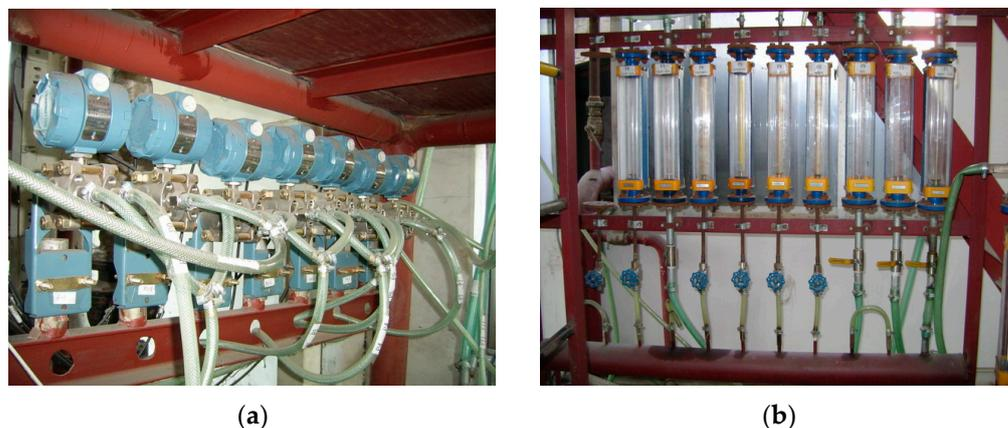
**Figure 3.** (a) Differential pressure transmitter image; (b) flow meter image.
