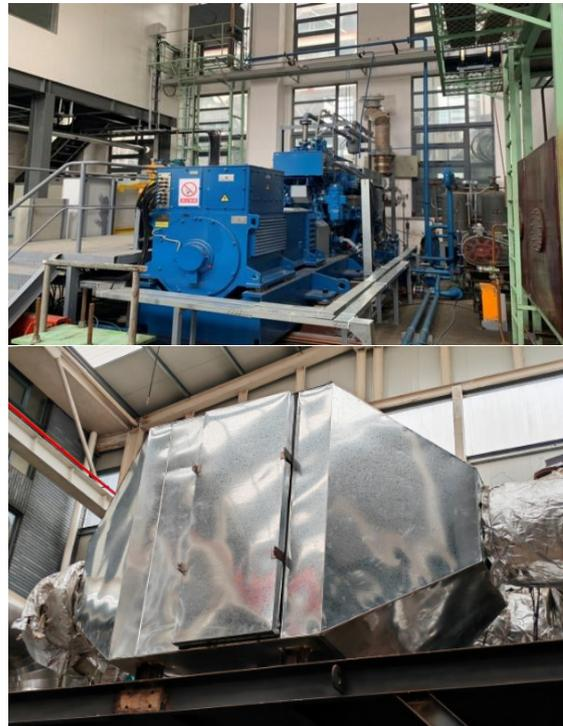
**Figure 1.** Wärtsilä 20DF Engine and DPF test system.
