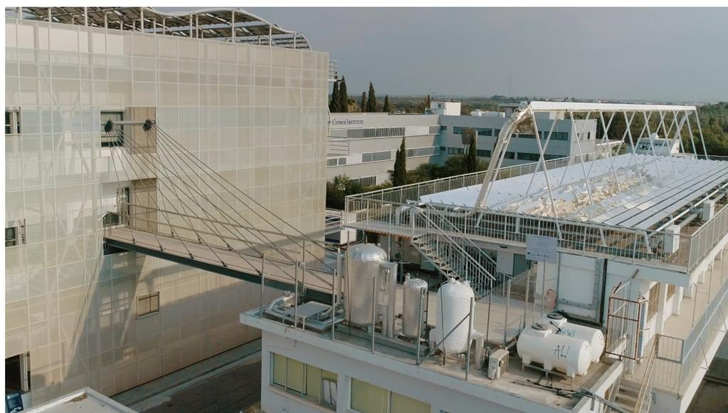
**Figure 1.** The Linear Fresnel Collector at the Cyprus Institute (right) and the Novel Technologies Laboratory [25] (left).
