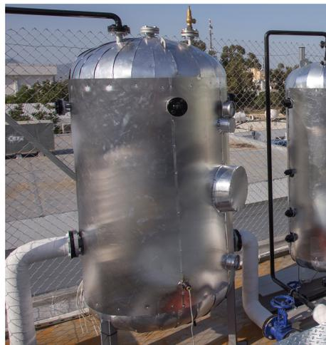
**Figure 4.** Buffer tank of oil with electric heaters wrapped around, allowing the expansion of the oil under pressure with Nitrogen gas.
