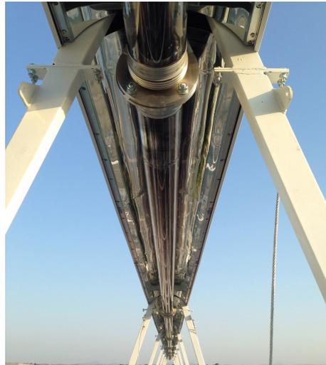
**Figure 3.** Receiver of the LFC, 32 m long with eight evacuated tubes in series.
