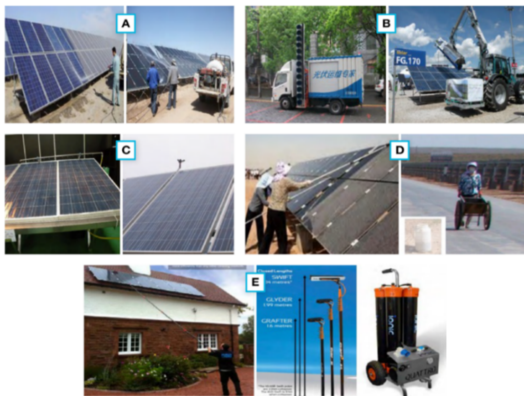
Figure 9. Popular PV panel cleaning methods in the desert. (A) Spraying water; (B) special cleaning vehicle; (C) water pipes; (D) human method; (E) special pressurized water brush.
