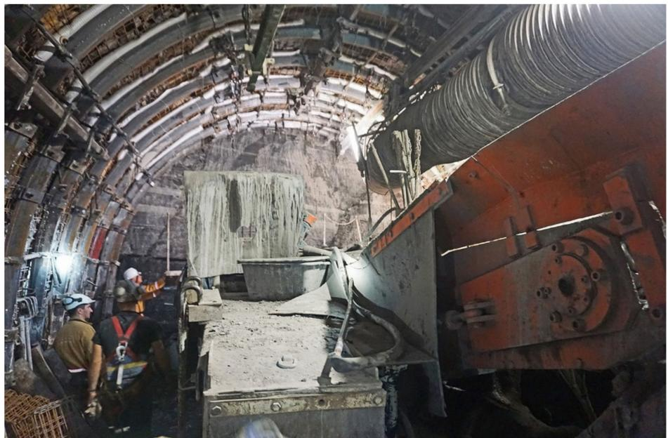
**Figure 2.** View of the mining face of a gallery drilled with a roadheader.
