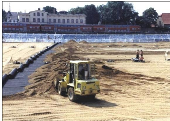
**Figure 17.** Reinforcement with aramid geosynthetics at the foundation level of the Gröbers junction 2001 railway embankment (sinkholes up to 4 m in diameter were present).
