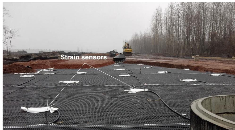
**Figure 4.** Second monitoring layer, measurement of elongation in geosynthetic reinforcement—Ruda Śląska, N–S route, Poland 2018 (example of monitoring application).
