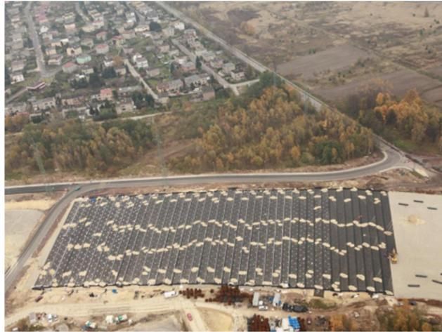
**Figure 16.** Reinforcement with aramid geosynthetics at the foundation level of the A1 Pyrzowice–Piekary 2011 motorway (shallow mining exploitation and mining faults).
