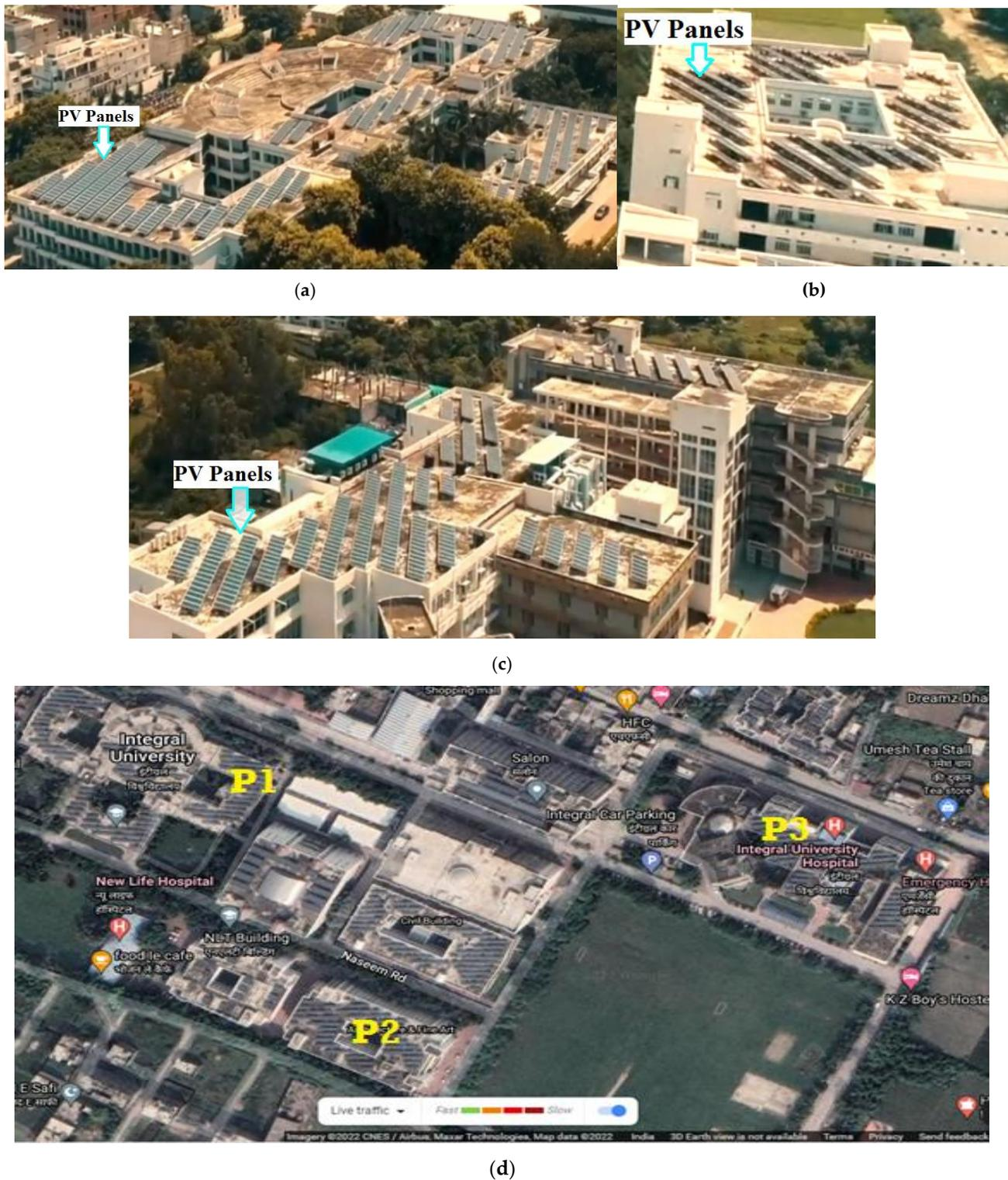
**Figure 3.** (a) 230.4 kWp Rooftop Solar PV System ( $P_1$ ); (b) 108.8 kWp Rooftop Solar PV System ( $P_2$ ); (c) 128 kWp Rooftop Solar PV System ( $P_3$ ). (d) Aerial view of the considered ( $P_1$ ,  $P_2$ , and  $P_3$ ) SPV Plant.
