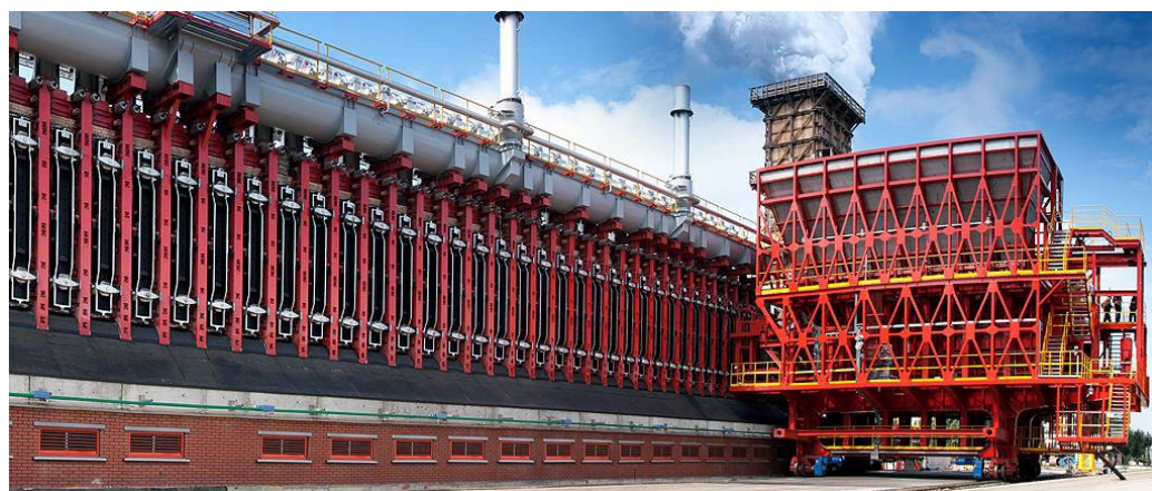
Figure 1. Stamp-charged coke oven battery at Coking Plant Czestochowa Nowa (Poland).
