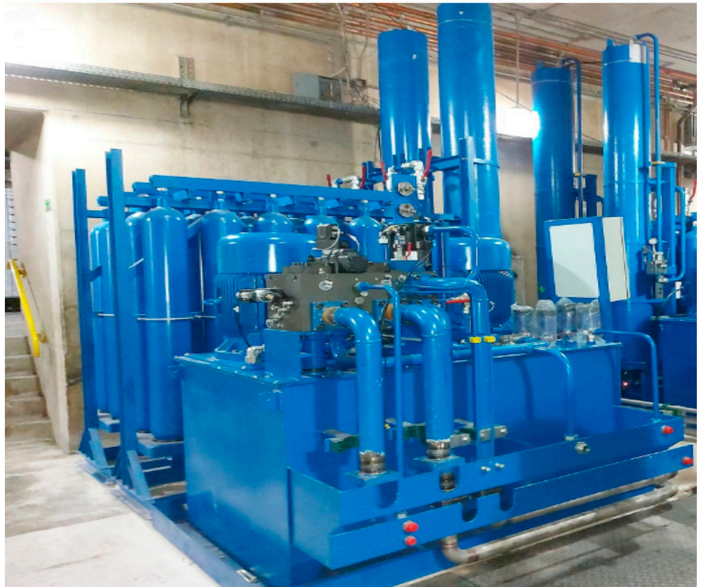
Figure 5. Hydraulic power unit of the speed governor.
