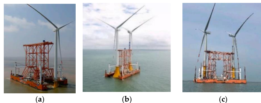
Figure 3. One step installation example of the composite bucket foundation. (a) Xiangshui wind farm (3.5 MW); (b) Dafeng wind farm (6.45 MW); and (c) Rudong wind farm (4 MW).
