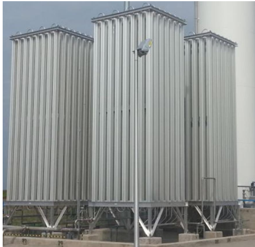
Figure 1. Block of four ambient air vaporizers in LNG regasification station.
