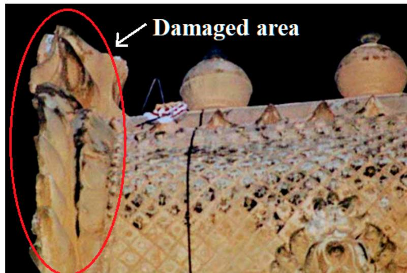
Figure 19. Keralanthakan gopuram damaged due to lightning strike.
