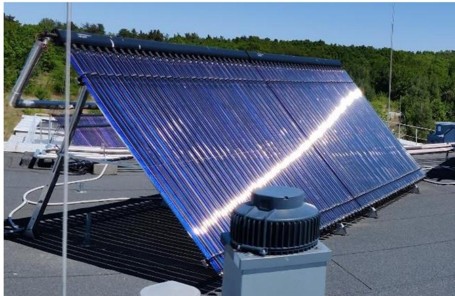
**Figure 3.** Kingspan Thermomax DF 400-30-way solar collector (60-way module).
