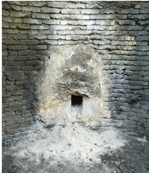
**Figure 3.** Ash deposition around the gas outlet duct leading to chimney S2 as observed during the kiln discharge procedure following carbonization Test 1.
