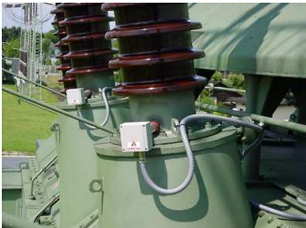
Figure 18. Crossing monitoring sensor [65].
