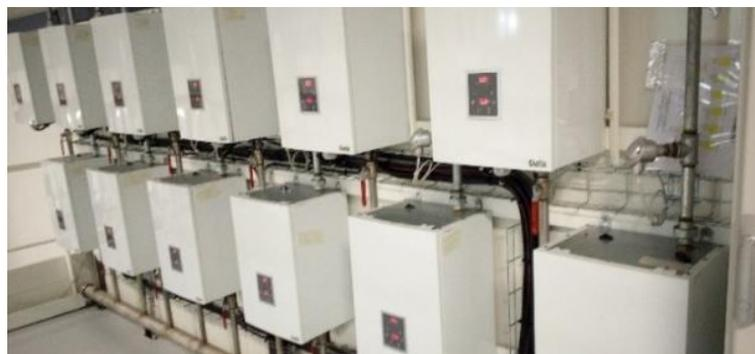
**Figure 8.** Electrical boilers.
